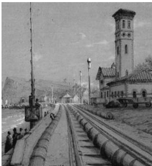
Telegraph wires sealed in atmospheric tubes alongside a railway track
